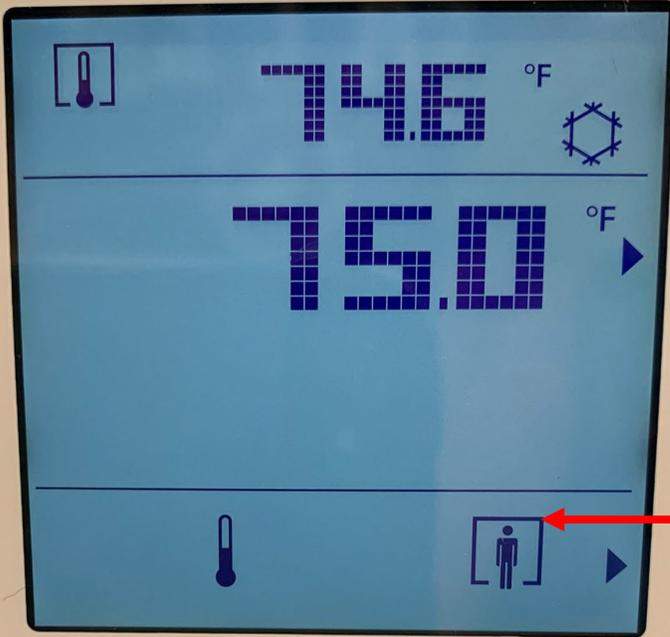
The person icon moved into the box indicating that the system has accepted the 4 hour call for cooling. After 4 hours, the room will stop cooling and the button will need to be pushed again.
